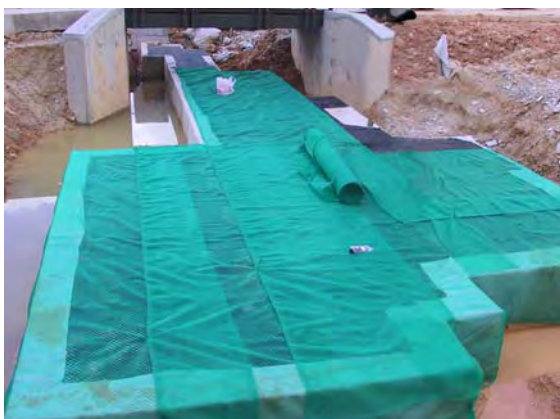
VersiTank® Infiltration System and the completed 'Rain Garden'
